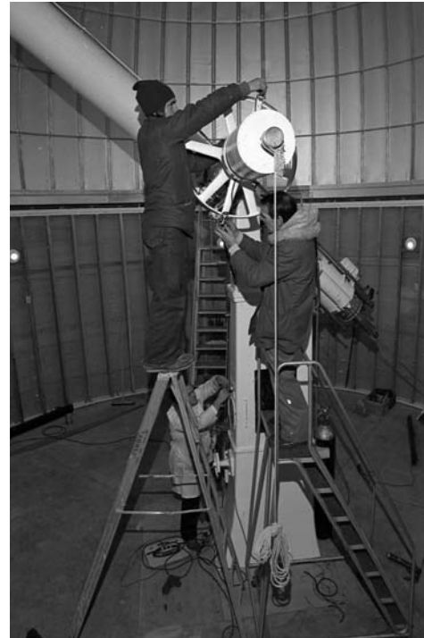
Because of the technical nature of its collection and the desire to demonstrate many of the artifacts, the Museum needed a large and highly skilled technical staff. Here, technicians install the telescope after it has been lowered into place through the roof of the observatory dome. Frank Askew, on the right, was an instrument-maker whose principle job was maintaining the telescope. (CSTM 75-639)
